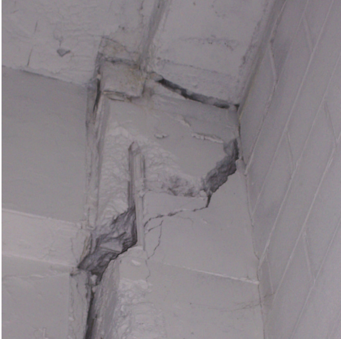
Enlarged view of the corner cracked column. The surrounding structure is covered and could not be observed.
