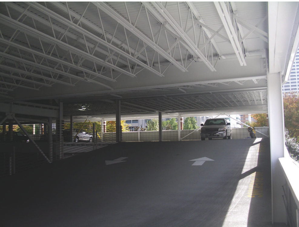
Throughout the garage, new joists were added in between the original joists to decrease the slab's span.
