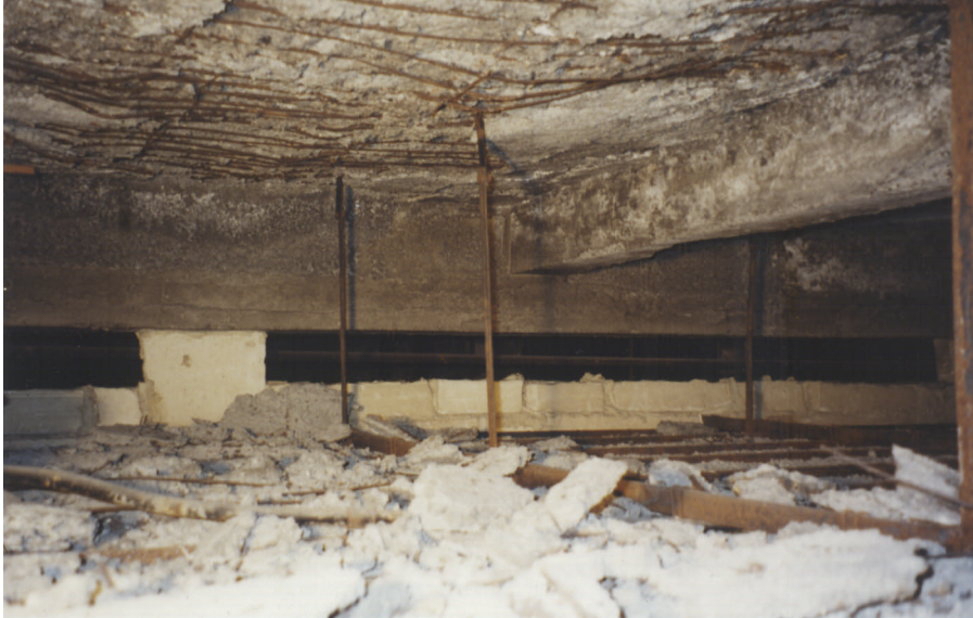
Chunks of the deteriorated cinder concrete roof slab landed on the flimsy stucco ceiling. The ceiling was hung from the same deteriorated roof slab.
