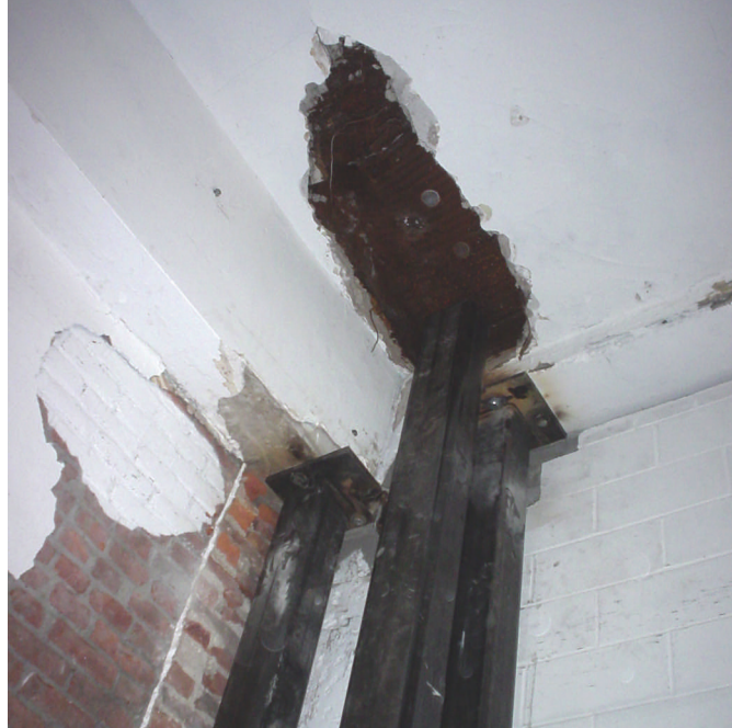
Hollow steel columns, 6 in. by 6 in., now reinforce the damaged concrete corner.
