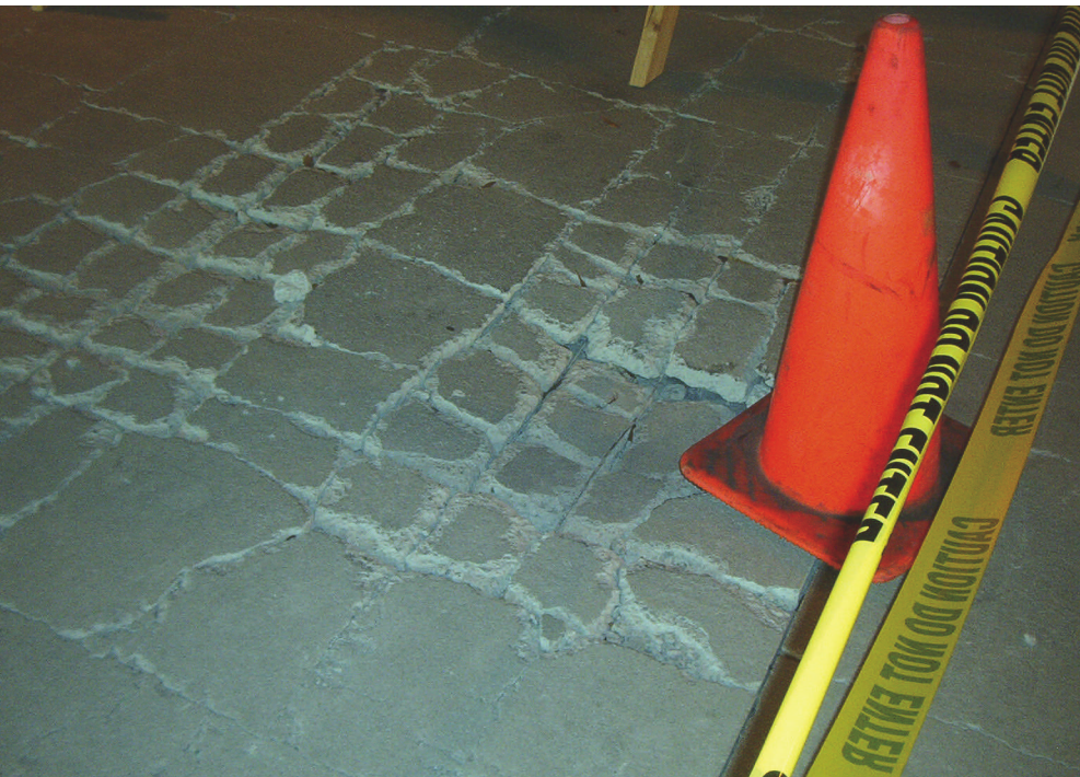
The original concrete slab was so badly cracked that it had punched through the deck in some places. Portions of the slab were barricaded.
